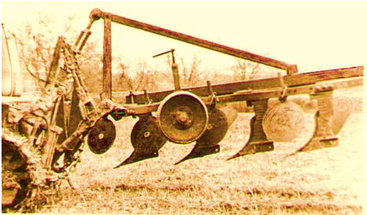
Fig. 1. A short-sized plow with inclined disc knives [9, 10]
